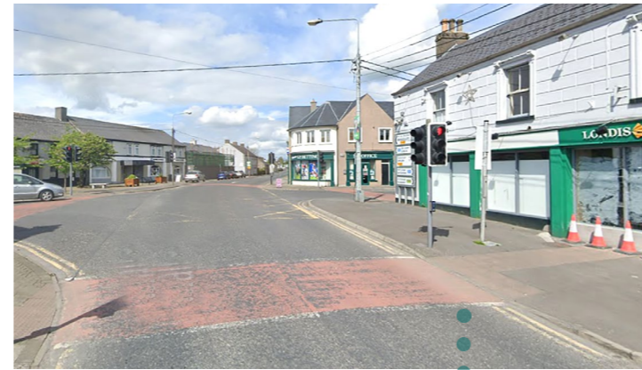
Above: Main Street Photo of Castledermot Main Street as existing.
