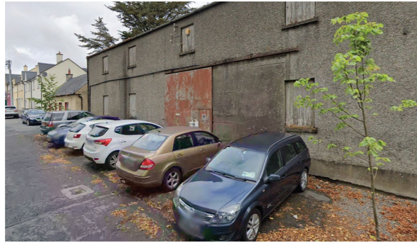
Above: Derelict site
