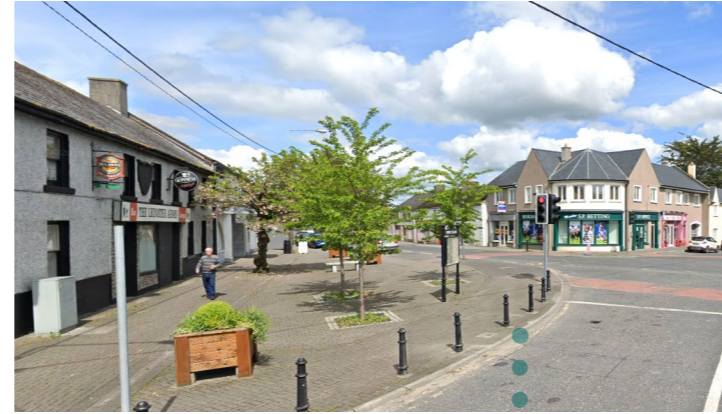
Above: Market Square Castledermot Photo of Market Square as existing.
